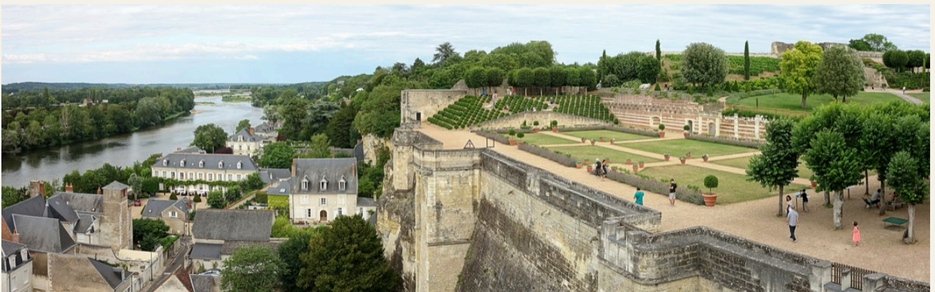
Amboise, the terrace above the river. The gardens sit on the platform of a far larger royal palace, most of which is gone. Photograph Velvet / Wikimedia Commons, CC BY-SA 4.0.
