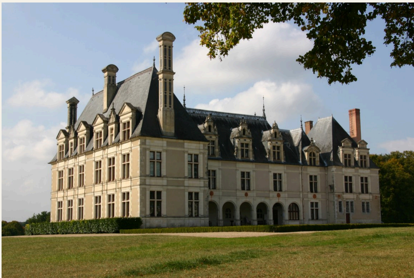
Beauregard, Loir-et-Cher. Identify the material first, then read the damage. Photograph Gerd Eichmann / Wikimedia Commons, CC BY-SA 4.0.
